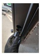
4 Remove the wire from the frame (if your door comes with a Smart Lock).
