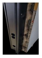
The casing and J profile must be installed flush with the edge of the frame.
