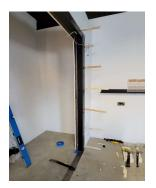
7 Check the level of the upper (horizontal) frame. If necessary, use shims for leveling.
