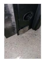
41 Rotate the square pin to adjust the drop seal. Adjust both the drop-down seals at the top and the bottom.
