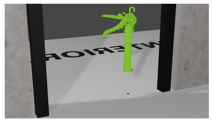
6) Install the socket on the floor hole by gluing it and screwing 2 buldex screws
